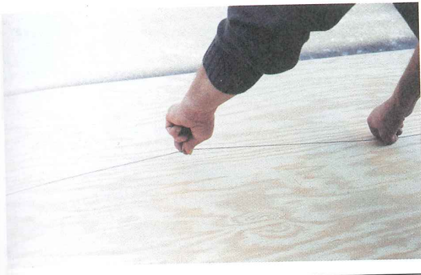
FIGURE 11-22 Snapping a chalk line.
